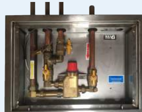
Sensor Probe installed on the outlet pipework of the TMV
